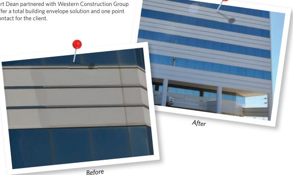
Stuart Dean refinished more than 35,000 square feet of the exposed architectural metal on the building's façade, including the application of protective coatings on these surfaces and the removal of sealants and gaskets. Stuart Dean also cleaned and re-polished all stainless steel window mullions on all elevations and added new stainless steel column base covers at the ground floor entrances.
